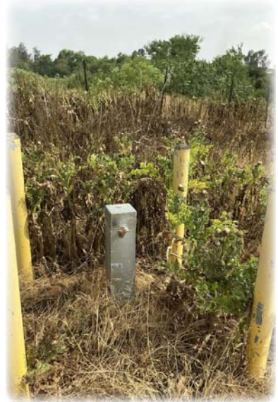
Prado Basin Monitoring Well
