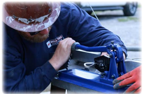
Cable Installation at the Pomona Extensometer Facility
